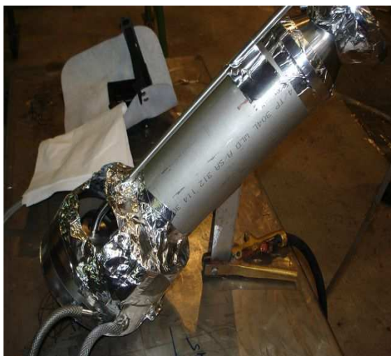
Photo 14: TIG welding of nozzles
