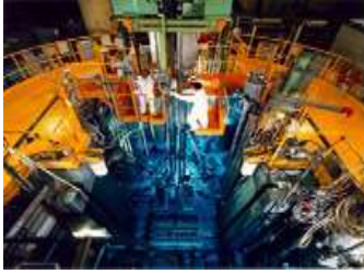
ORPHEE neutron beam research reactor.
