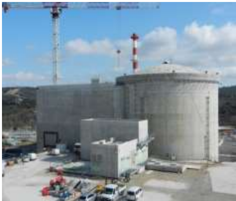
JHR Building site- Mid 2017
