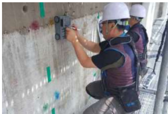
FIG. 7. Rebar scanning to avoid cutting existing rebar
