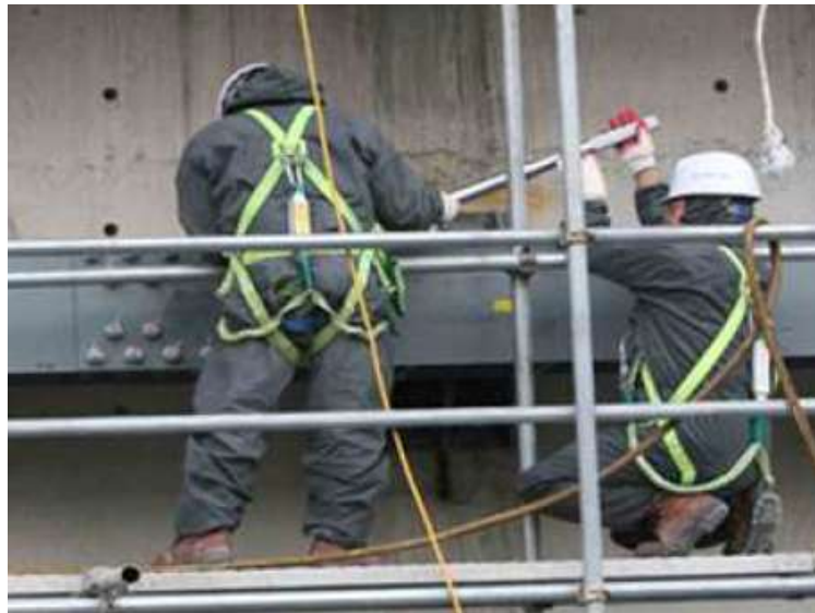
FIG. 12. Workers are tightening the high-tension bolt with regulated torque.
