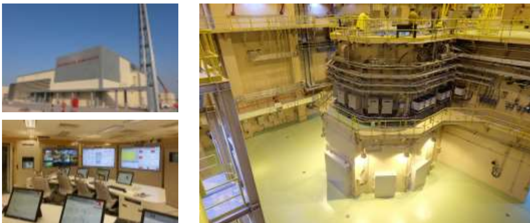
FIG. 4. View of reactor building, main control room and reactor hall of JRTR.
