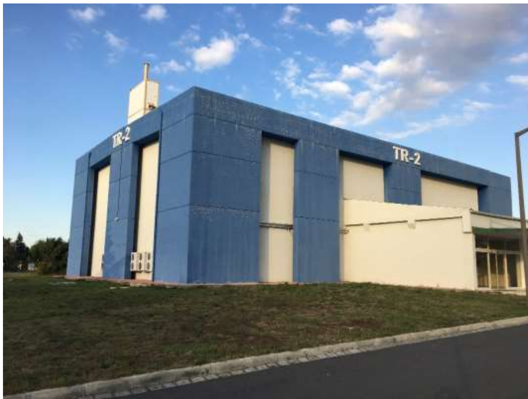
FIG. 2. TR-2 Reactor building after reinforcement
