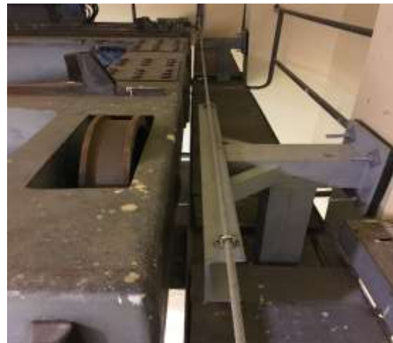
FIG. 7. Crane buffers
