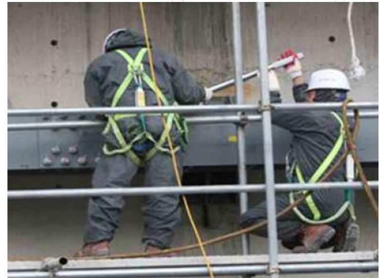
Workers are tightening the high-tension bolt with regulated torque.
