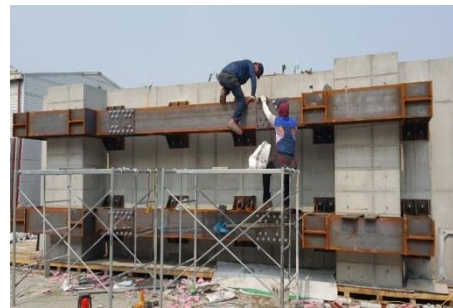
Arrange anchor bolt using template, Size inspection of built-up section, Assembling of built-up section, Relocate the specimen
