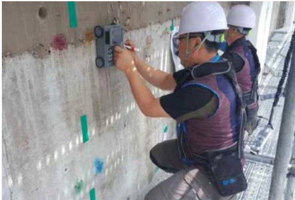
Rebar scanning to avoid cutting existing rebar
