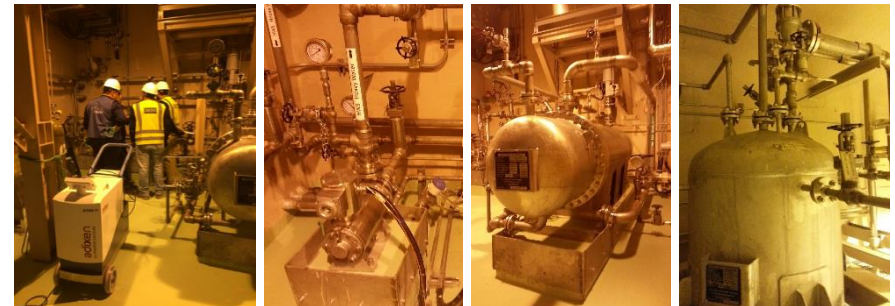
Leak test HWS Pump / Heat exchanger / Expansion tank
