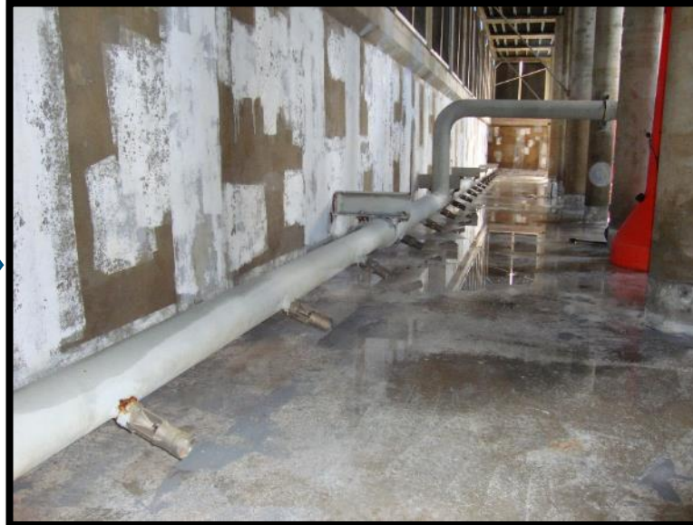
Patchwork Basin coating
