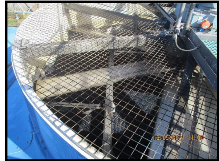
SS Frame, Installed
