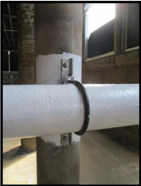
Submerged Pipe-support
