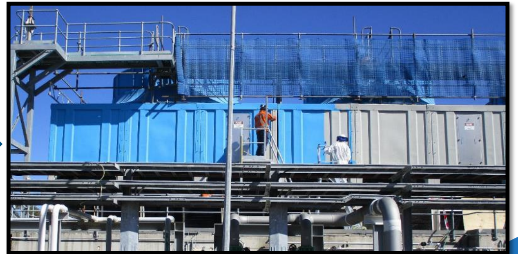
Paint Application: Undercoat (Grey), Topcoat (Blue)
