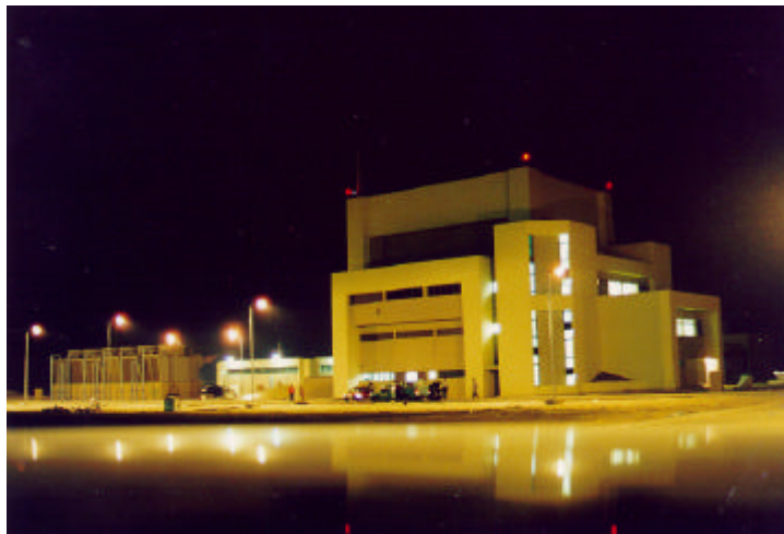
Fig. 1 ETRR-2 General View
