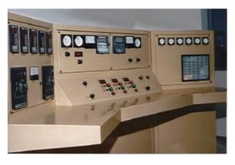
Figure 4. The IPR-R1 Reactor New Control Console
