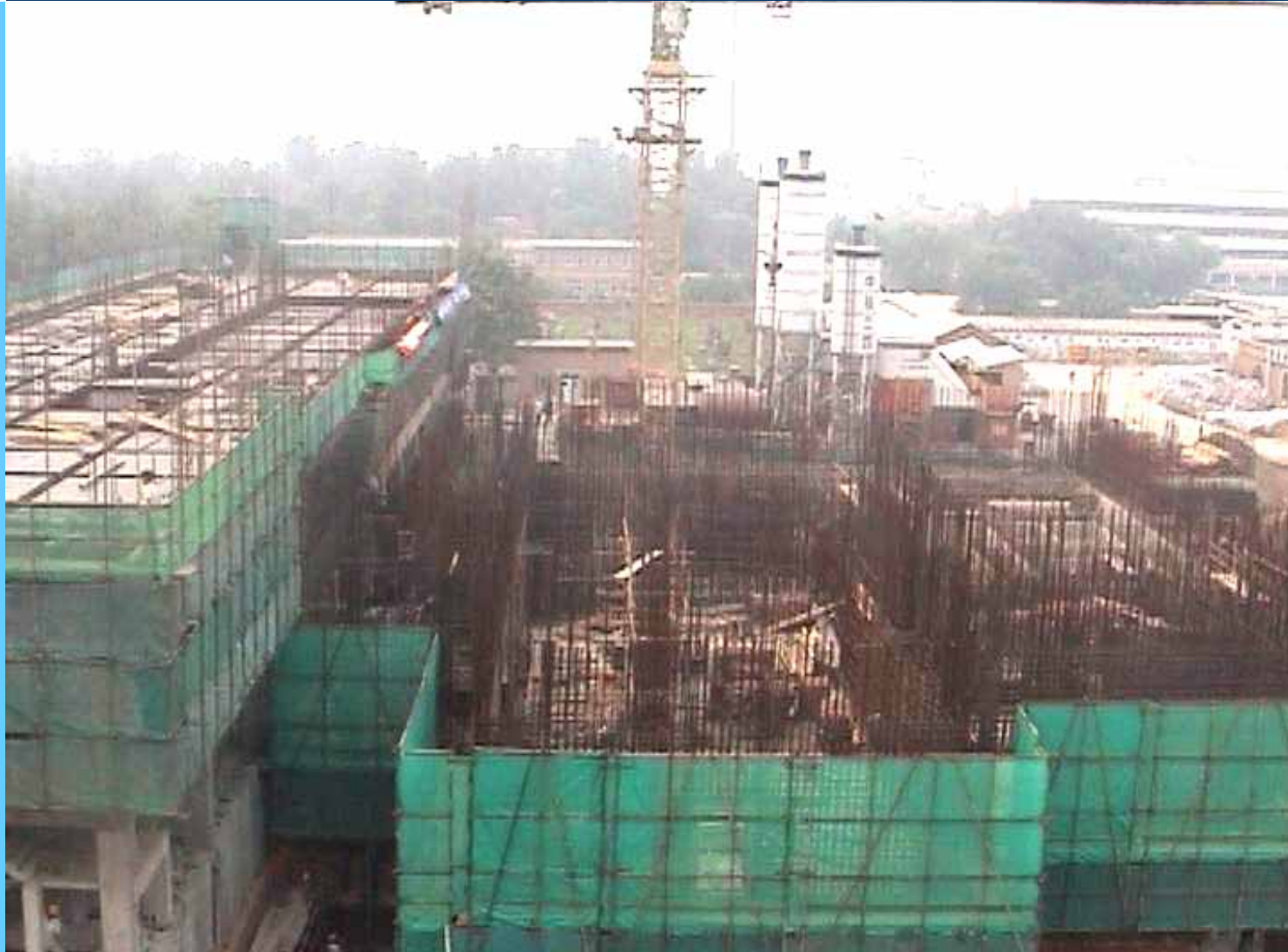
Full view of CARR site
