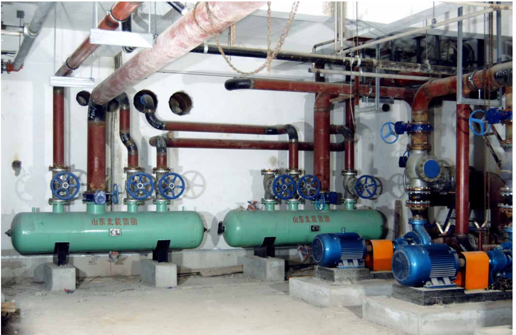
Piping system installation of 03 sub-item( 2005.7)
