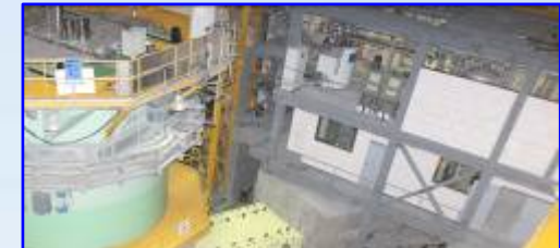
System Commissioning on Schedule & the 1st Cold Neutron in Sep. 2009
