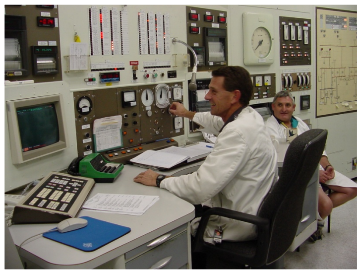
HIFAR Control Room
