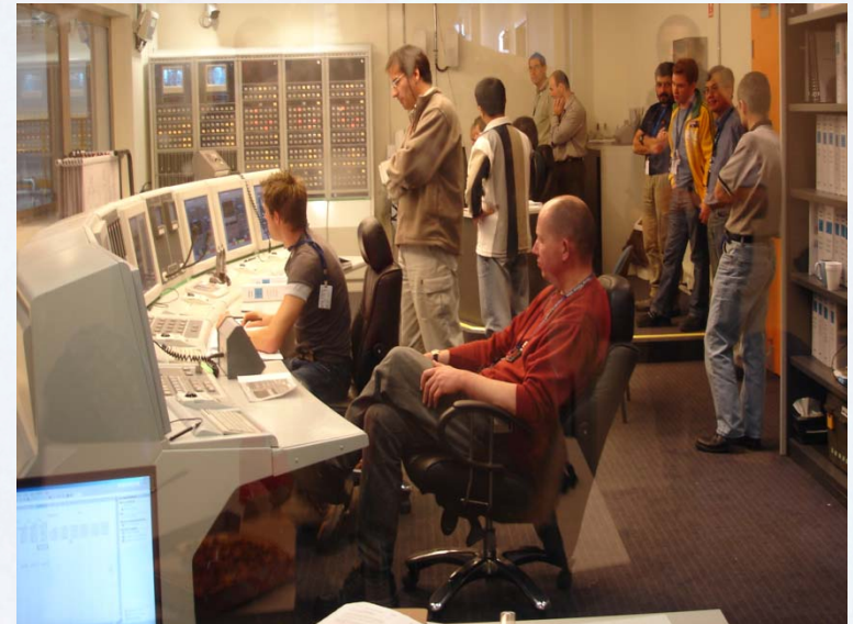
During Reactor commissioning
