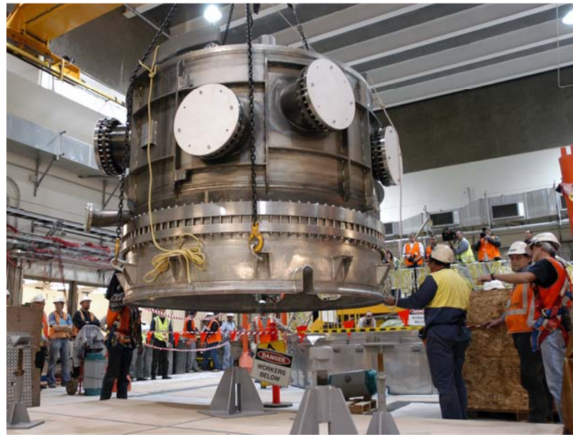
Reflector Vessel – during installation
