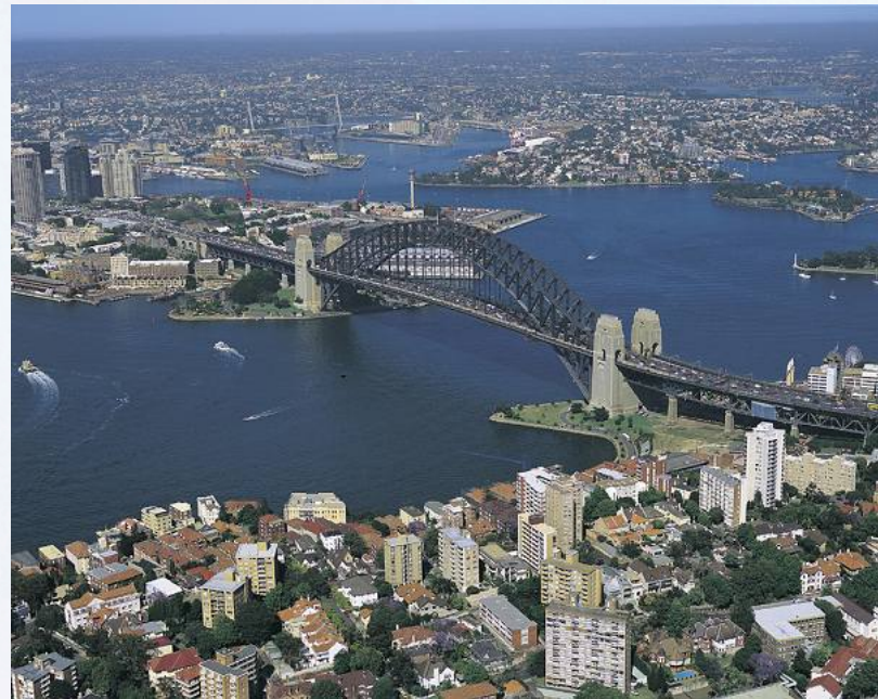
Sydney Harbour Bridge
