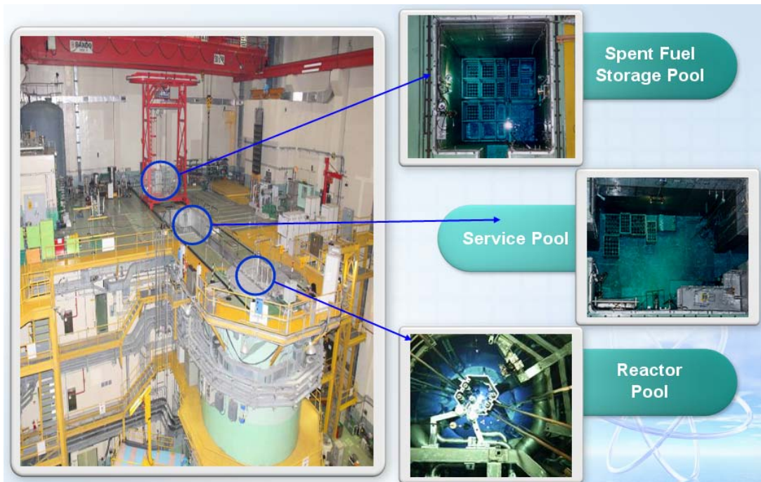
Fig. 2 Arrangement of Pools inside the Reactor Building
