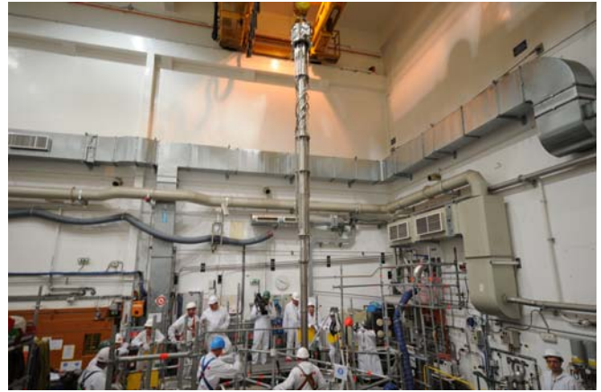
Fig 2 : CABRI introduction of the new pressurised test section
