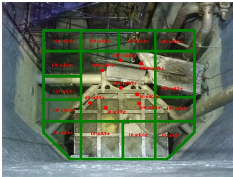
Fig 3. Radiation dose rate map of the reactor pool when completely drained
