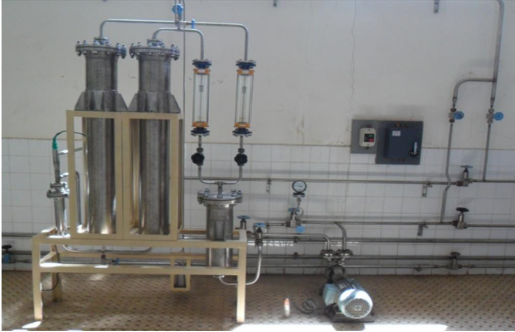
Fig.4.11: Reactor pool water purification system
