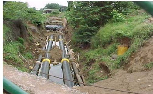
UG lines after weathering protection
