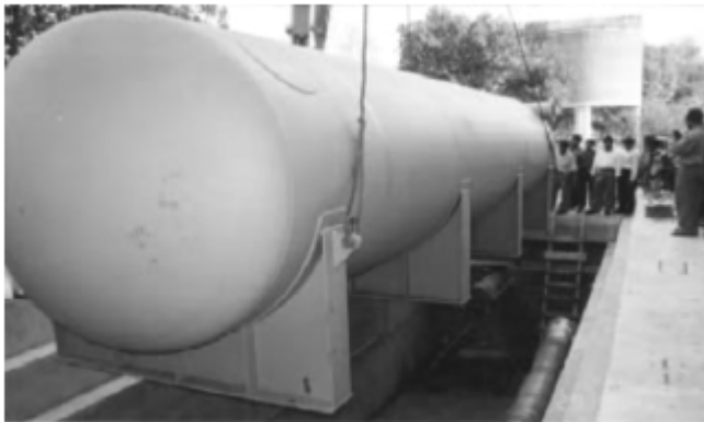
Fig. 2 New N-16 decay tank with aluminum saddle Fig. 3 Piping arrangement around H/E
