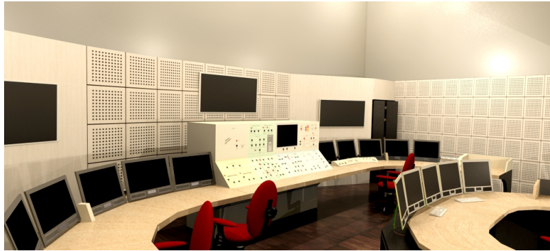
Fig. JHR Control room
