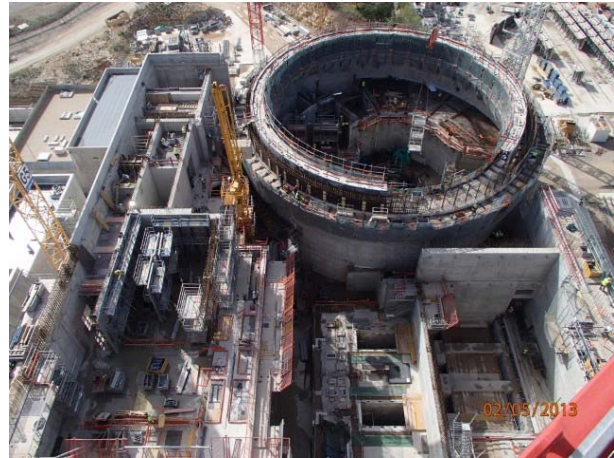
Fig 2. Overview Reactor Building (copyright CEA)
