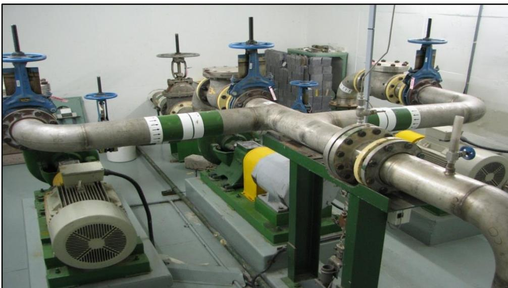
**Figure 3 : Pump Room, Showing the Emergency Core Cooling Pumps (the two outer pumps) and the Decay Heat Removal Pump (the middle one)**
