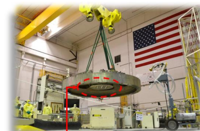
ATR's vessel head being lifted into place after CIC with new top head closure plate installed
