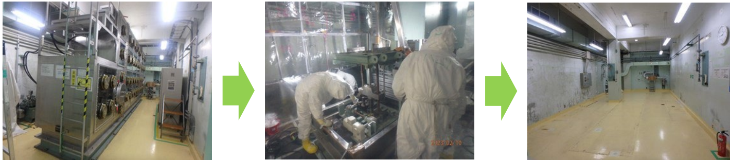
Example of equipment demolition (glove box)
