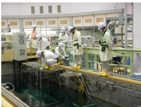
Storage work after removal of control rods
