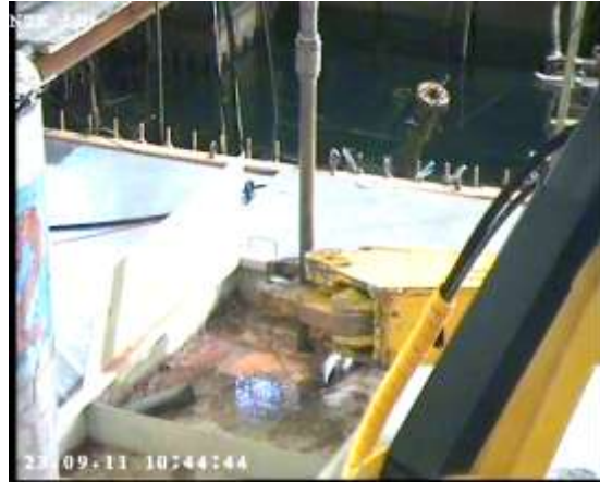
Fig. 3. Cutting and fragmentation of channels using BROKK robotics
