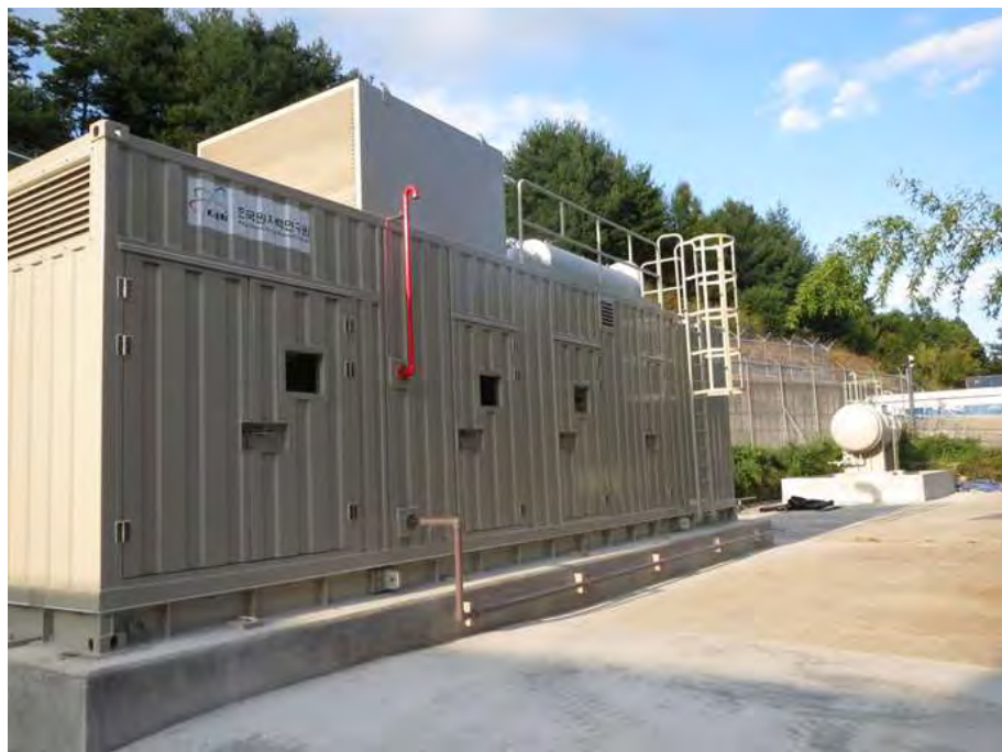
Fig 3. Extra DG and Fuel Storage Tank
