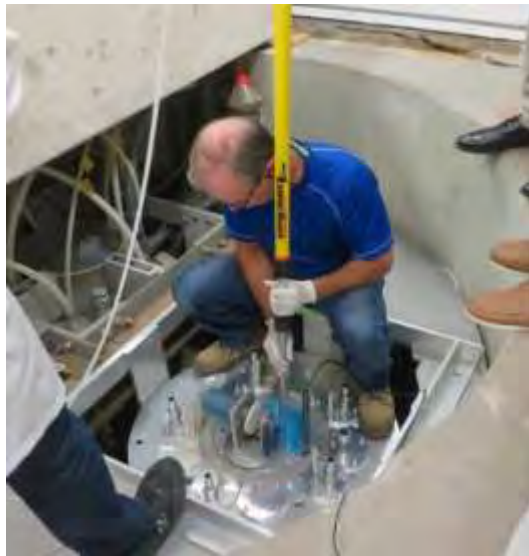
Figure 4 - Shim removal process
