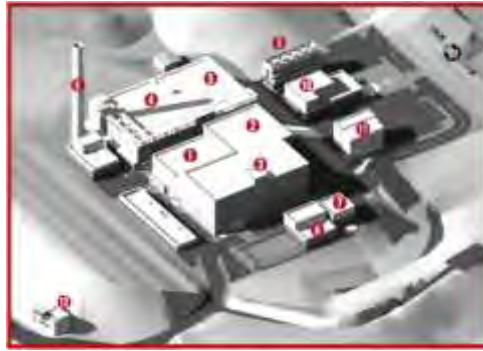
Fig 3. Elevated view of the site; 1) FMPF, 2) reactor facility, 3), utility facility, 4) RWTF, 5) RPF, 6) electric building, 7) diesel generator building, 8) stack, 9) cooling tower, 10) demi water system and pump house, 11) natural evaporation building, 12) guard house
