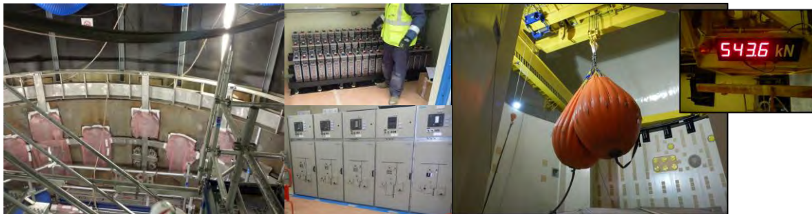
Support structures for the pool liner, electrical cabinets and batteries, Polar crane Test
