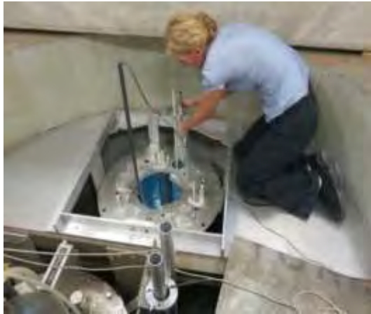
Figure 3 - Top plate assembly with support beams
