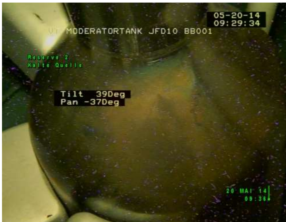
Figure 5: CNS inside moderator vessel after 10 years of operation in May 2014
