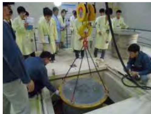
Fig 3. Exchange of Thermal Column for Exp-6
