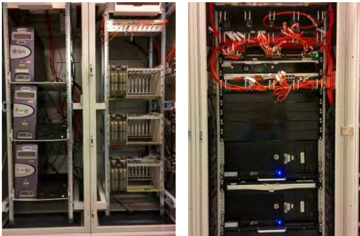
Fig 1. Comparison of the old (left) and new (right) equipment cabinets. The shift to the use of conventional IT hardware is very clear.
